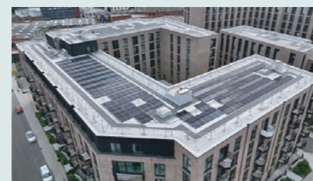
NOVEMBER: Solar Panels installed at our Leicester site
