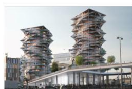
Kaktus Towers, Copenhagen SEK 1 334 M *
